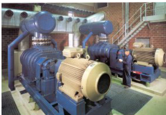
Application with a compressor
